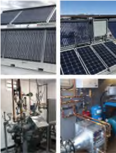
Figure 2: TISR® infrastructure for solar heating (Solar Collectors) and waste heating (blower heat exchanger) applications.
