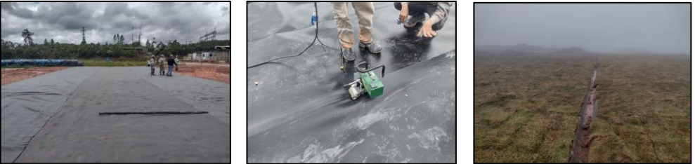
Figure 5 and 6 – Application of the geomembrane and completion of the work
