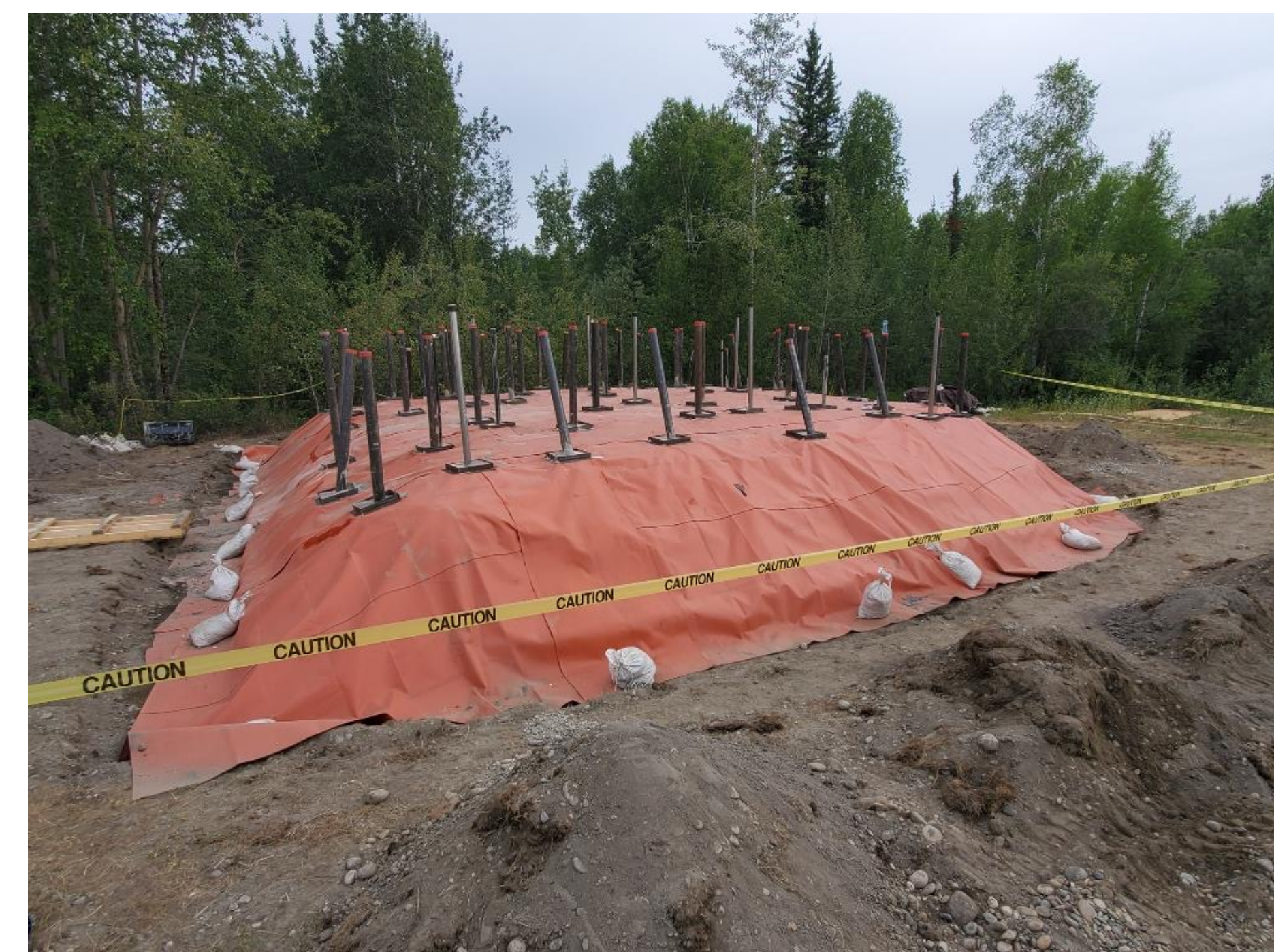
In-place treatment of PFAS-impacted stockpiles to avoid transportation and destruction.
