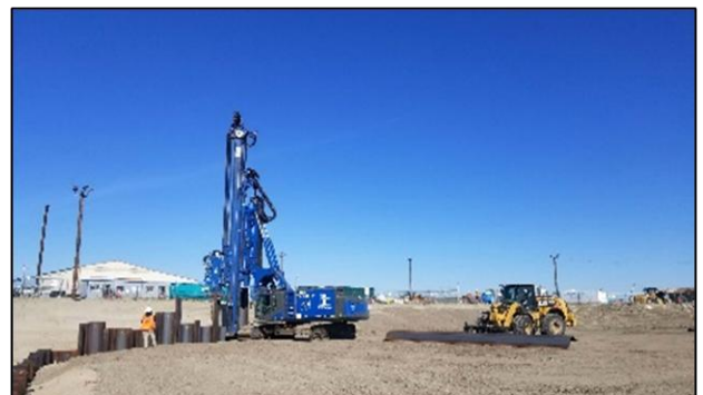
ABI Mobile Ram installing sheet pile.
