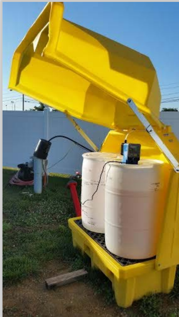
Recovery Well with Temporary Iron Precipitation Control
