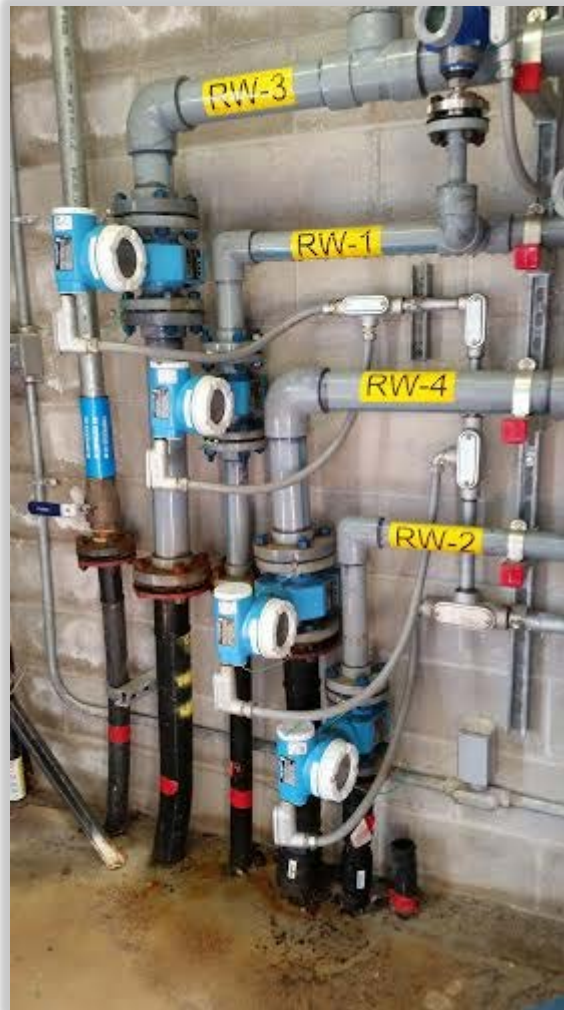
Recovery Well Flow Meters & Controls
