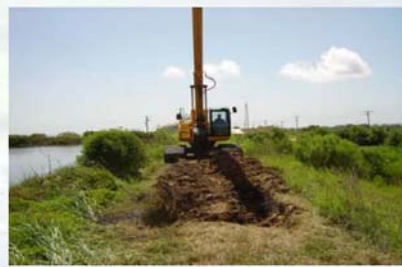
2 - A small pit was excavated in the berm beside the excavator to contain the sludge sample.
