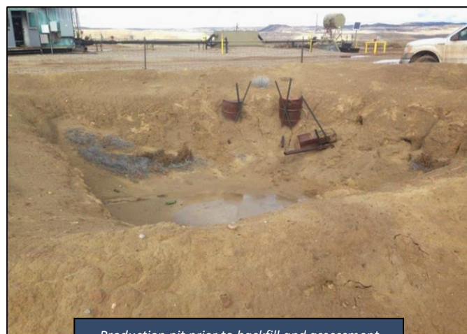
Production pit prior to backfill and assessment
